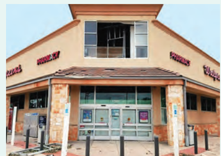
This Walgreens store in Texas was damaged in Hurricane Harvey.
